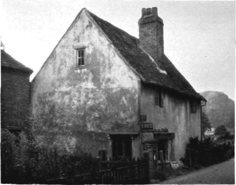
North-east view of the Darenth house, shortly before its demolition.
